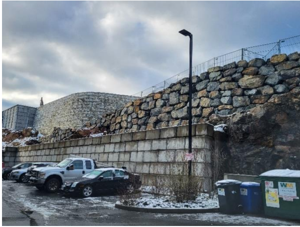
Four types of retaining walls facing multi-family development
