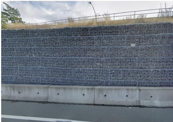
Gabion basket retaining wall with roadside jersey barriers
