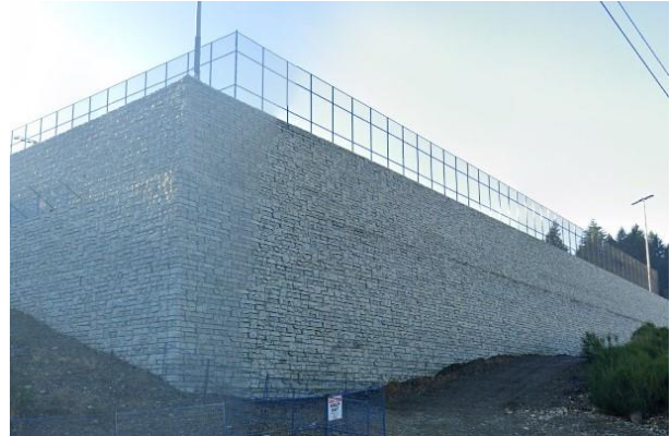
Large precast wall, one terrace, no landscaping
