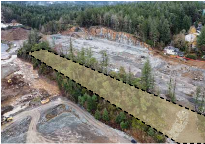
Overlay for discussion purposes only. Please refer to siteplan for accurate boundary line.
