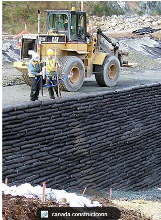
Typical MSE Installation
