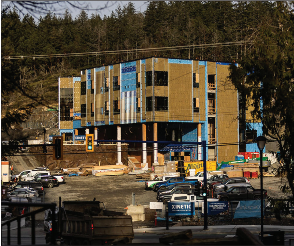
Construction continues on the new SCIANEW STELITKEL Elementary School in Langford. (Arnold Lim / Goldstream Gazette)
