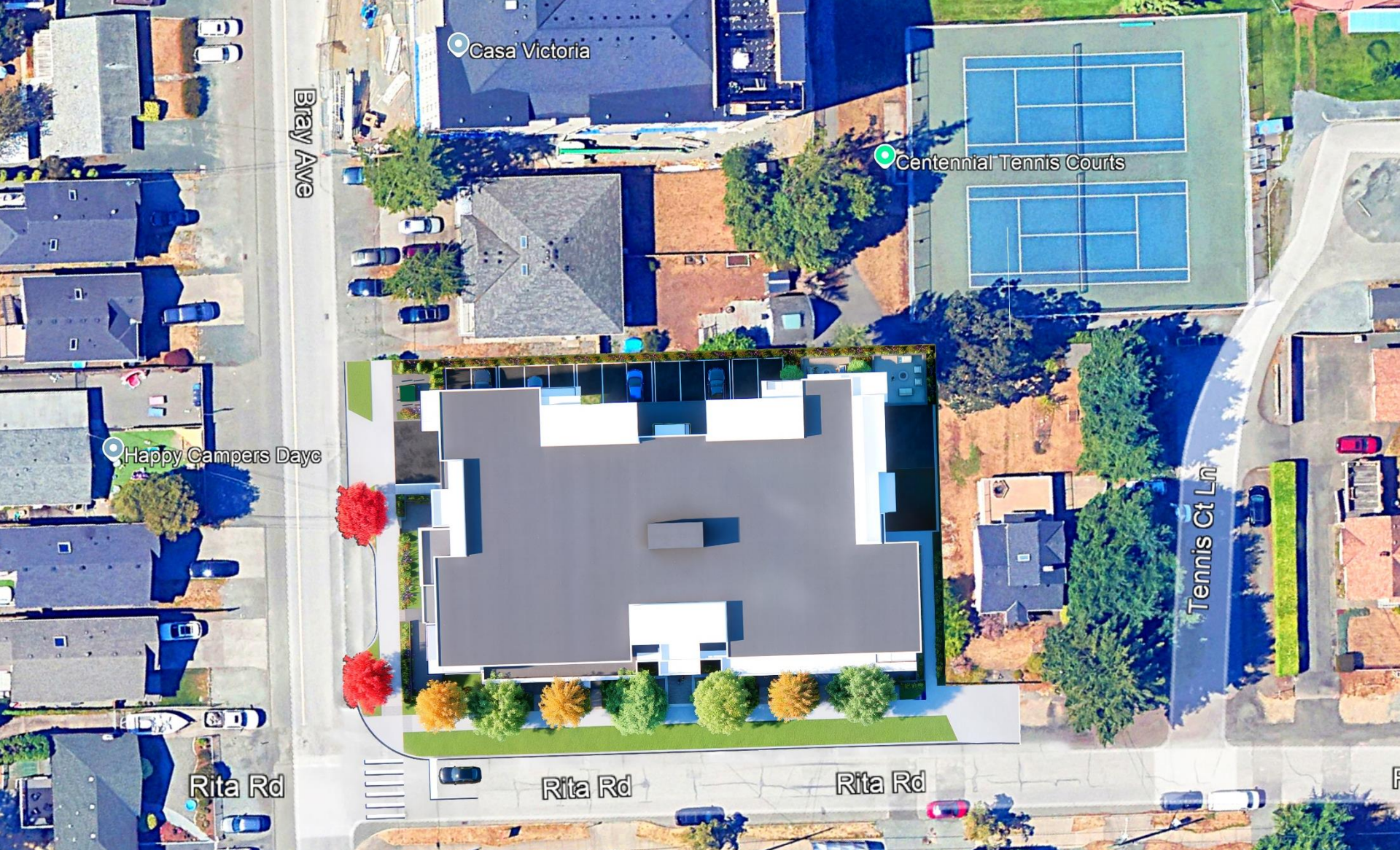
Development creates sidewalk off Bray down Rita towards Tennis Court Lane
