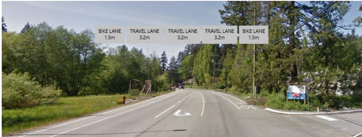
Figure 1: Latoria Road Typical Existing Road Cross-Section
