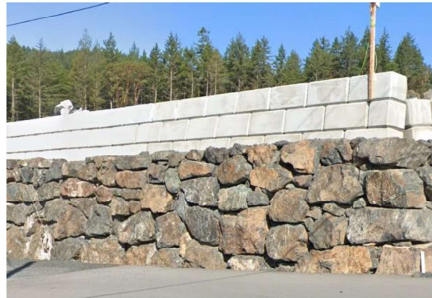
Lock blocks on top of boulder-stack (non-face mortar)
