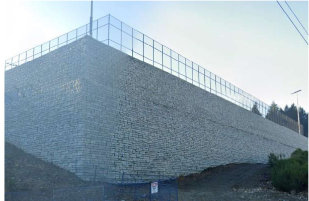
Large precast wall, one terrace, no landscaping
