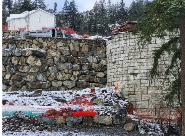
Two types of retaining walls facing collector road
