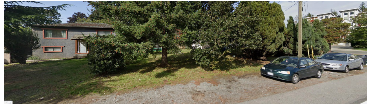
Strathmore Road View
