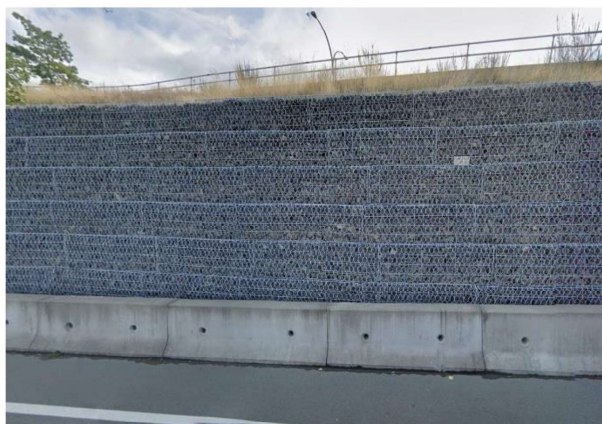
Gabion basket retaining walls with roadside jersey barriers
