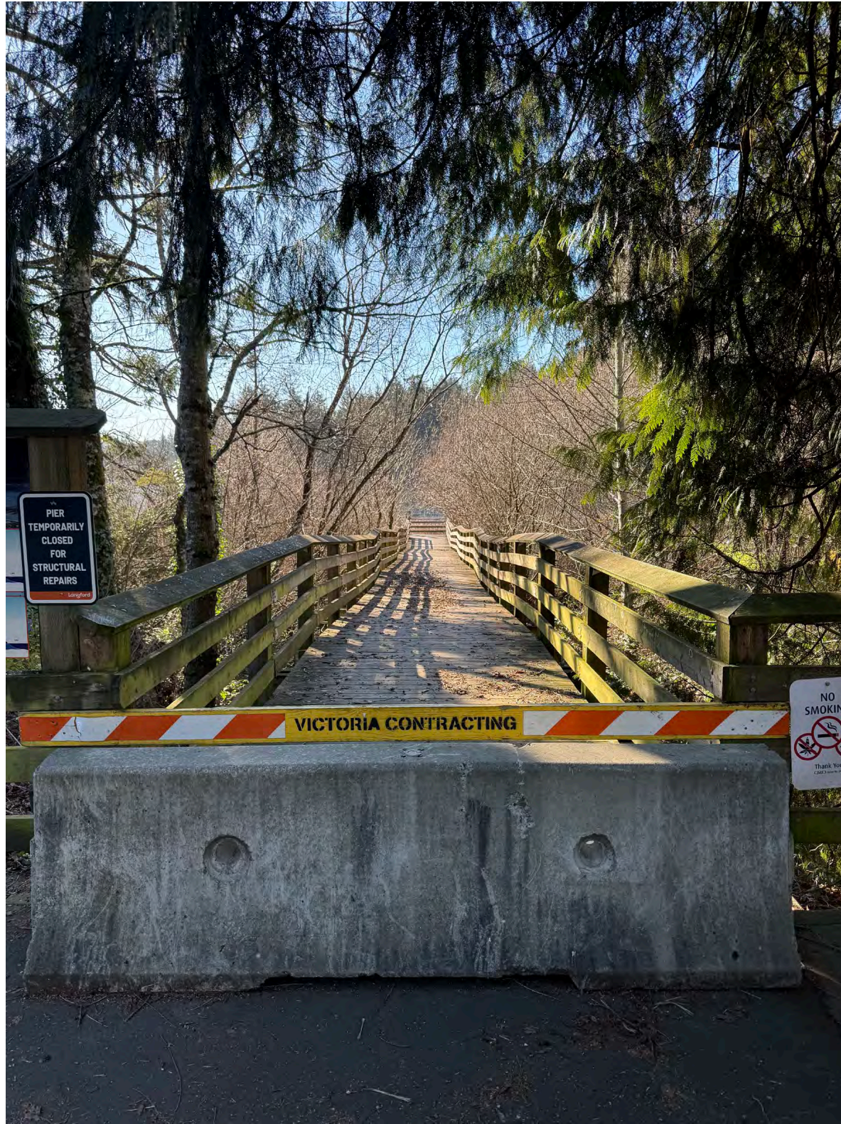
Florence Lake Pier Repairs
