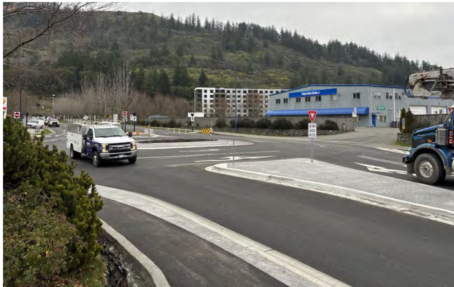
Amy Road at West Shore Parkway Roundabout Improvements
