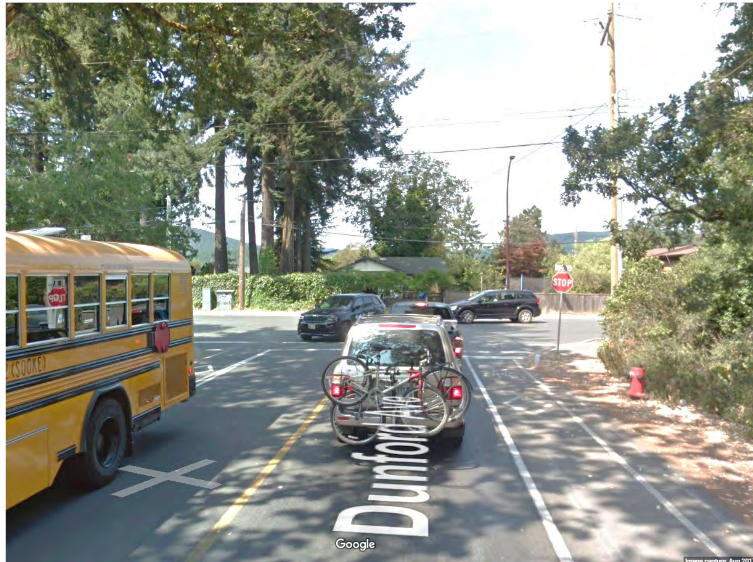
Traffic Signal at Leigh Rd and Dunford Ave
