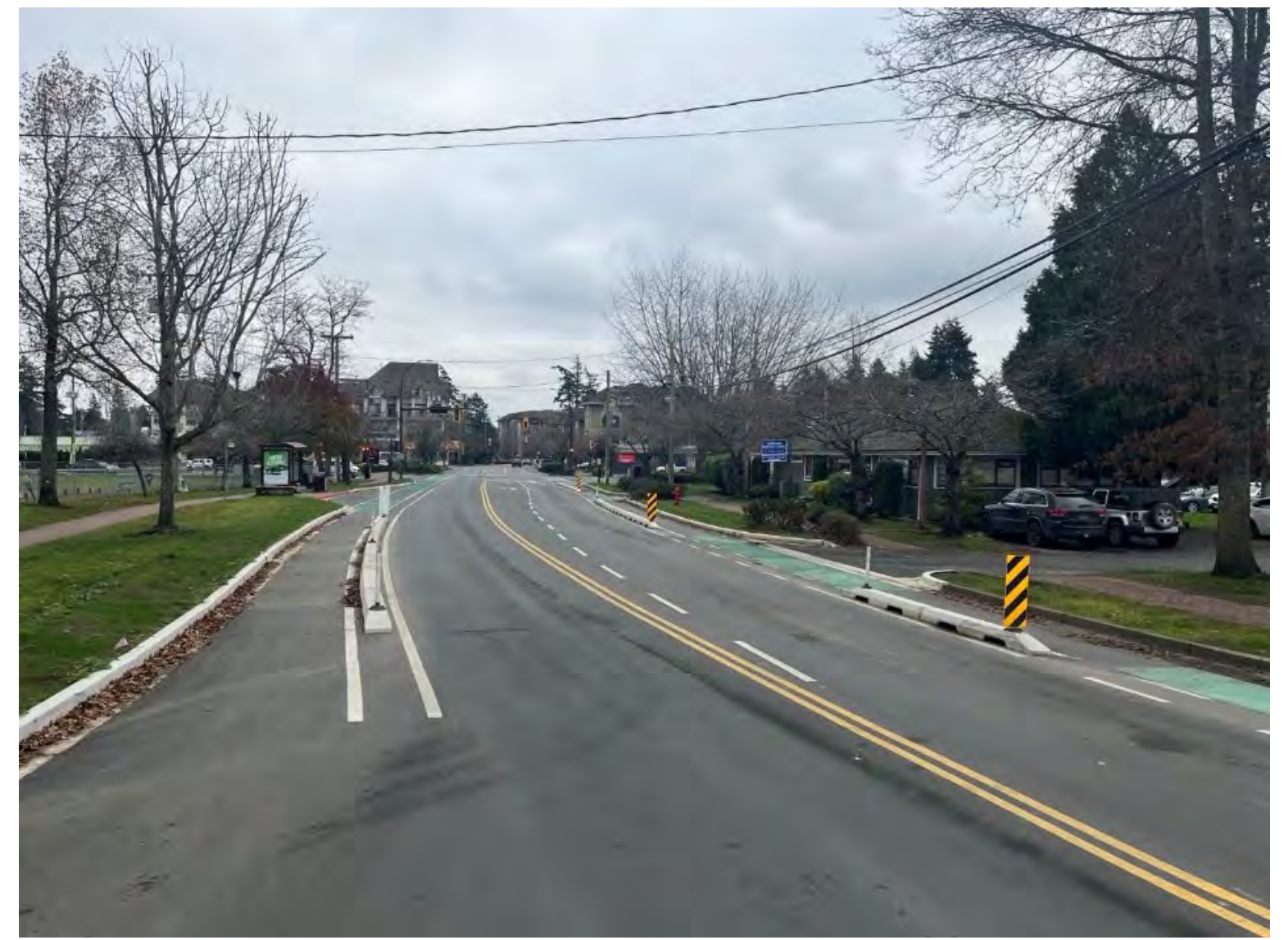
Goldstream Ave Protected Bike Lanes and Pavement Rehabilitation
