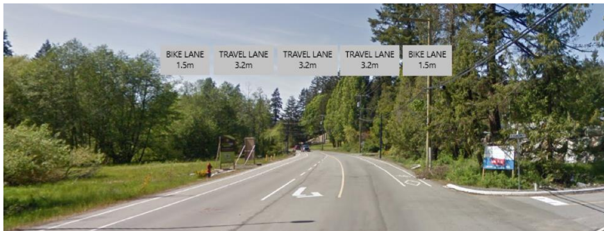
Figure 1: Latoria Road Typical Existing Road Cross-Section
